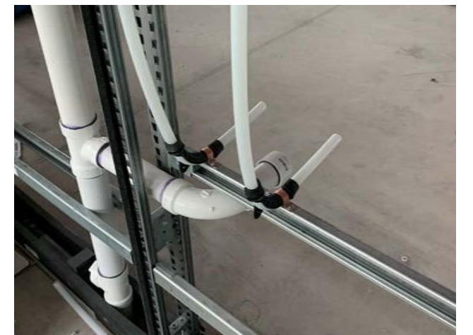
SINKS + MILLWORK ATTACH TO CLADDING WITHOUT ADDITIONAL BACKING
