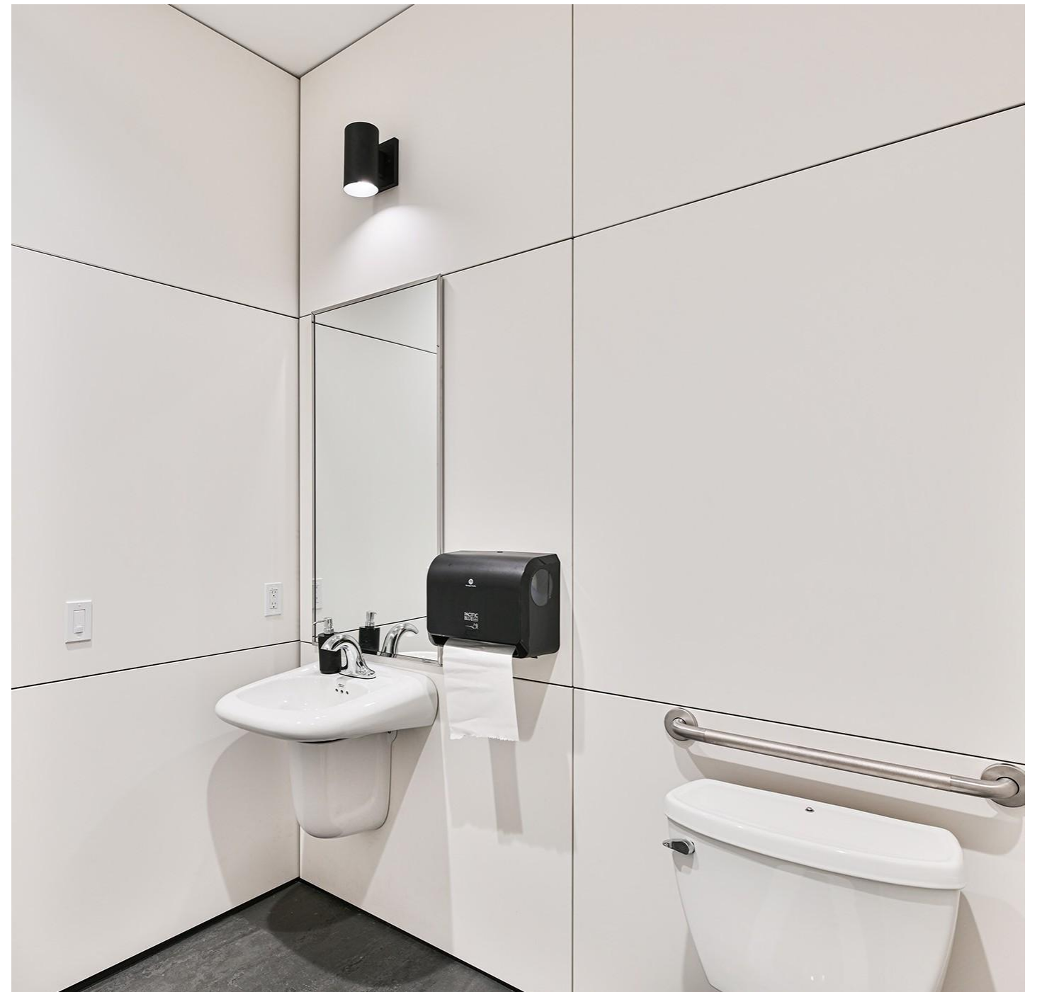
SINKS + MILLWORK ATTACH TO CLADDING WITHOUT ADDITIONAL BACKING
